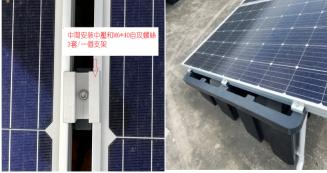
Fix the panels on the trays by 3pcs\*aluminum mid clamps and end clamps with 6\*45 screw. (if it's over 40mm width panel, should use longer screw)
