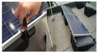
Fix the panels on the trays by the plastic end clamps with 6\*30 screw
