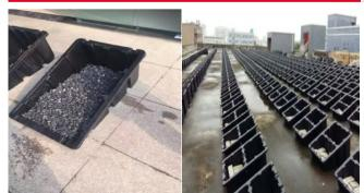
Put the plastic trays on the ground with gravels or stones(the weight should be 60-100kg per tray)
