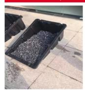
Put the plastic trays on the ground with gravels or stones(the weight should be 60-100kg per tray)
