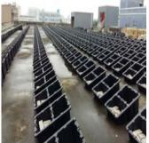
Put the plastic trays on the ground with gravels or stones(the weight should be 60-100kg per tray)
