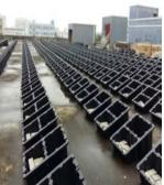
Put the plastic trays on the ground with gravels or stones(the weight should be 60-100kg per tray)
