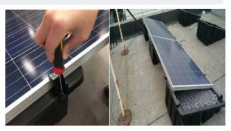
Fix the panels on the trays by the plastic end clamps with 6\*30 screw
