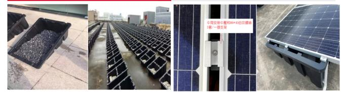
Put the plastic trays on the ground with gravels or stones(the weight should be 60-100kg per tray)
