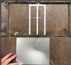
Insert the SpeedFlash® Shield fully as shown.
