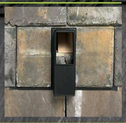
12 To hold the SpeedFlash® in place, use the metal spring support. Insert support via the bottom opening, hooking the support onto the cut under slate.
