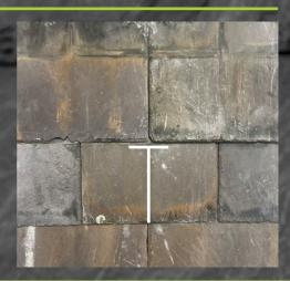
To conclude the line drawings for cutting purposes, measure 37.5mm / 1.48" left and right from the centre of the rafter line. Draw vertical lines from the 190mm / 7.5" horizontal line, down to the bottom of the slate.
