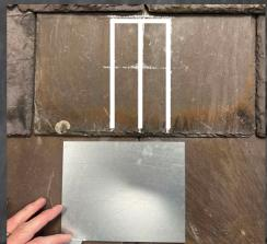
Insert the SpeedFlash® Shield fully as shown.
