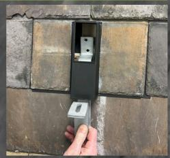
14 Insert foam at the bottom opening of the SpeedFlash®.
