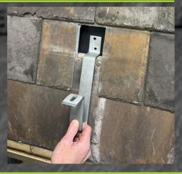
9 Use shims / packings to create clearance between the bracket and the roofing material.
