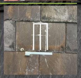
6 Now you have cut the top slate(s), you need to cut the lower course to create the working area (the area in which the bracket will be fixed).
