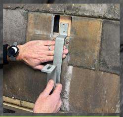
10 Cut down SpeedFlash® to required size (determined by the size of the slate).
