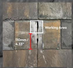
Using the angle grinder, cut out the 'working area' on the slate i.e. the area from the 110mm / 4.33" horizontal line and the 190mm/ 7.5" horizontal line.
