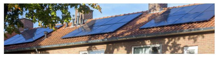
The SolarEdge solution includes a single power optimiser with four Maximum Power Point Trackers (MPPT) for harvesting more energy from each panel. Each MPPT connects to one or two 60-cell panels or one 72/96-cell panel, and works exclusively with the new SolarEdge single phase inverter with compact technology. The inverter is extremely compact, easy to install, and is available in 1kW, 1.5kW, and 2kW sizes.
