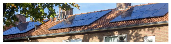
The SolarEdge solution includes a single power optimiser with four Maximum Power Point Trackers (MPPT) for harvesting more energy from each module. Each MPPT connects to one or two 60-cell PV modules installed on the roof and works exclusively with the new SolarEdge single phase inverter with compact technology. The inverter is extremely compact, easy to install, and is available in 1kW, 1.5kW, and 2kW sizes.
