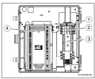
Fig. 28 Arrangement of components in the electric box
