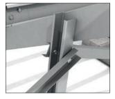
Fig.9 – Braces fit both sides of upright
