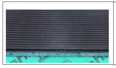
23) Fit 2 Bottom flashing hooks per panel
