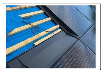
Fitting an External LHS flashing as shown
