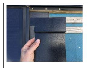
2) Fit Internal corner joining plate
