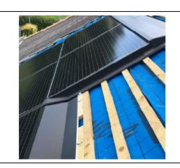
To Fit an external RHS flashing as shown
