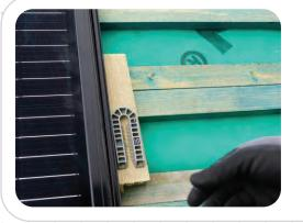
B: Over hang screw over batten in upper / middle part of panel
