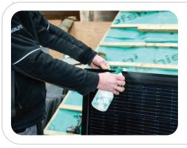
A: Use soapy water sprayed or applied to top seal to lubricate & aid fitting
