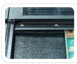
C: Fit 150mm section of expandible phone tape under frame of upper panel
