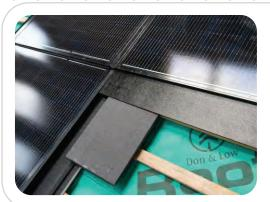
D: Fit Metal Bottom flashing or flexible bottom as standard
