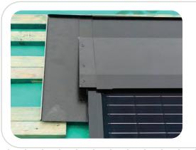
Push Top LHS Flashing **under** the top flashing
