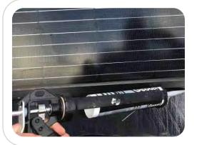
Apply very small bead of silicone on bottom edge of panel
