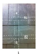
After locating the battens B1 & B2 and rafter position with the metal detector
