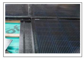
**3)** Fit additional panels around the corner and fit LHS flashing flashing
