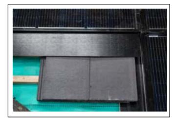
4) Fit metal bottom flashing or flexible bottom flashing as standard
