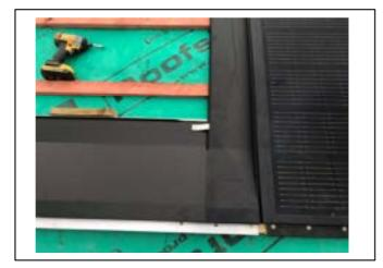
4) Slide RHS external flashing into place
