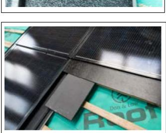
**3)** Fit 150mm section of expandible phone tape under frame of upper panel
