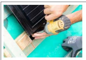
16) Fix panel with 6 screws per panel Don't let the panel drop or slip down as it will not be square
