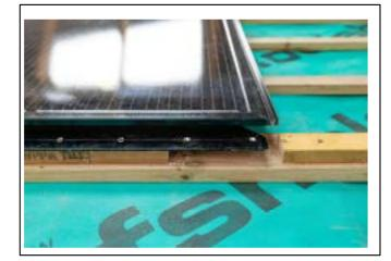
2) Cut out 200mm of top batten from RHS outside edge of panel
