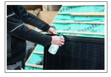
25) Use soapy water sprayed or applied to top seal to lubricate & aid fitting
