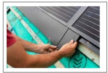
47) Slide Bottom flashing joiner into position
