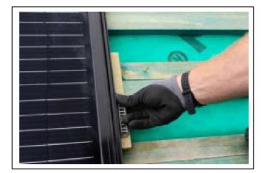
43) Slide panel support into position Parallel with RHS panel frame
